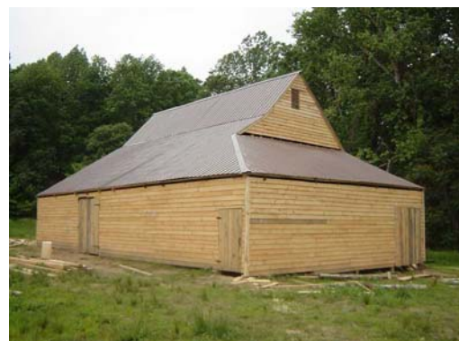
Barn restored with appropriate roof and siding.
