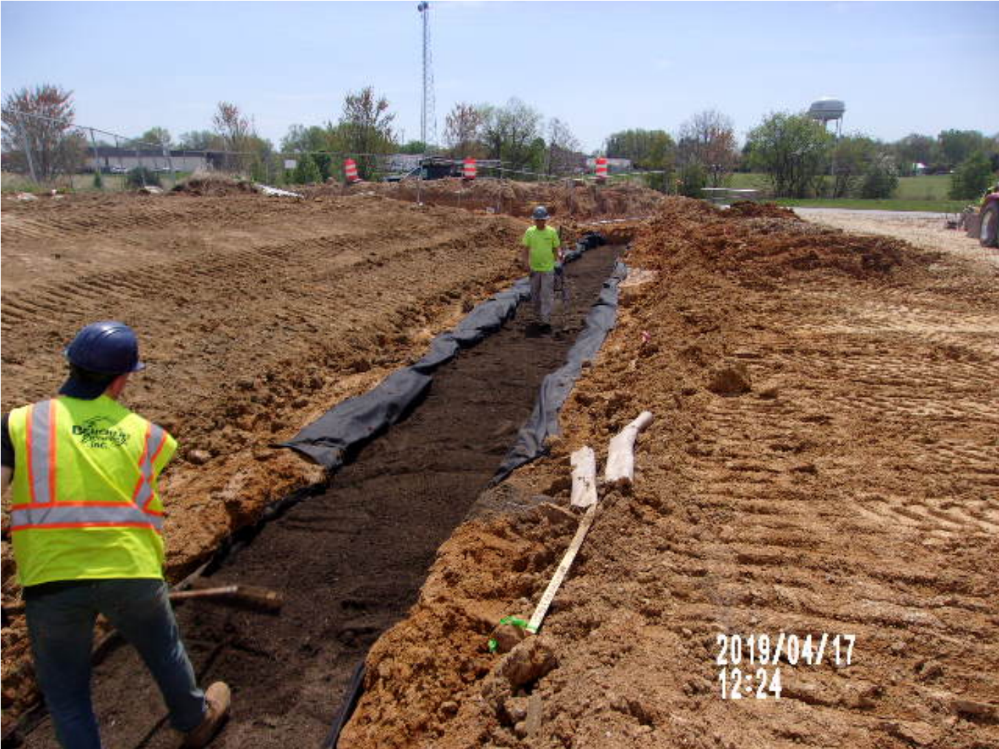
Installation of Bio-swale Near Main Entrance
