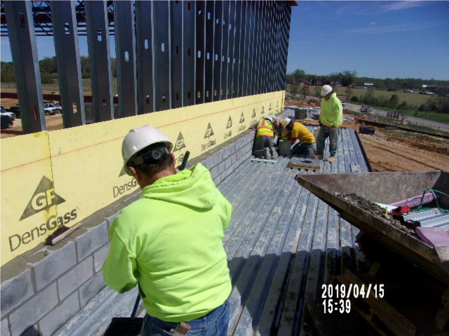
CMU Block Instillation on Library Roof
