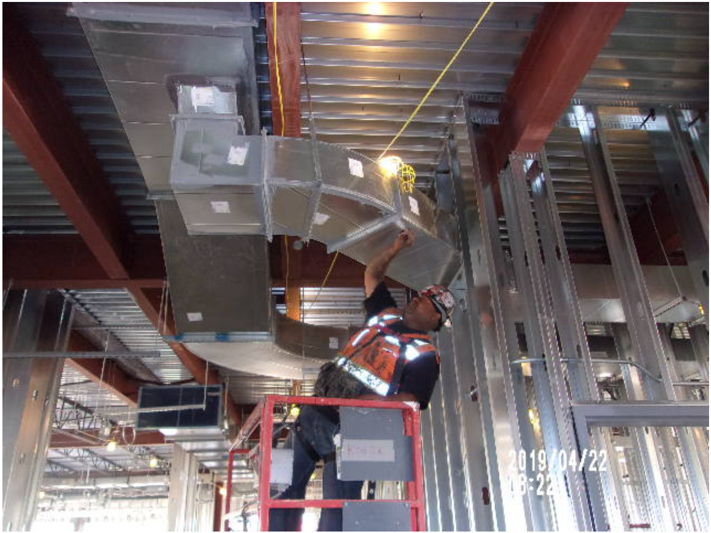
Installing Ductwork on Main Garvey Hallway
