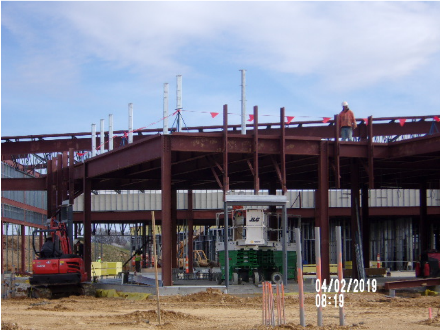
Screen Wall Installation on Library Side
